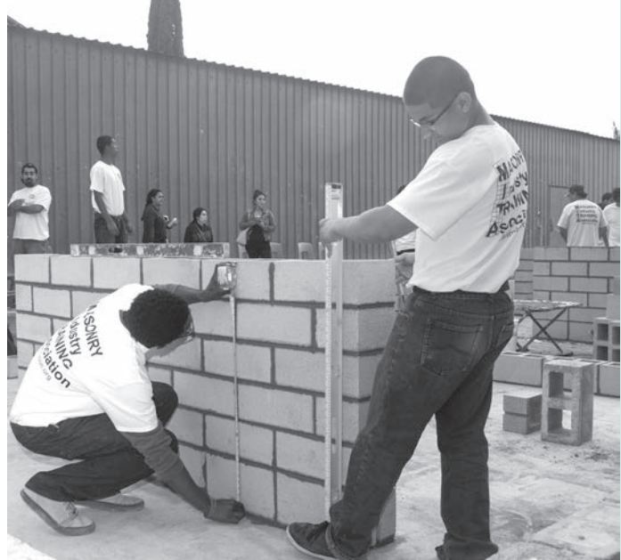
BUILDING TOGETHER: Jahsi and Emilio measure the dimensions of their long wall at the Top Notch Trowel competition. The two Boys Republic Masonry students earned second place for their structure.
